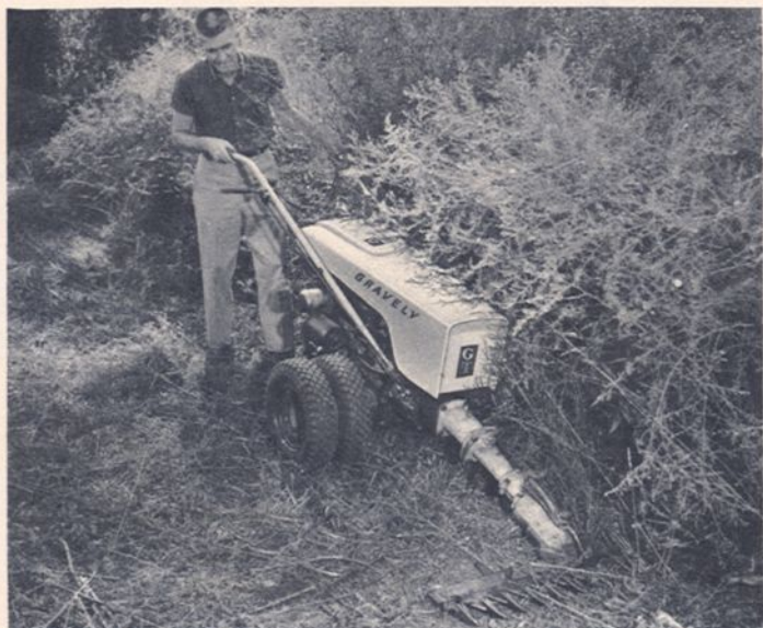
Gravely Sickle Mower cuts anything small enough to get between the guards . . . even saplings, weeds, brush!
